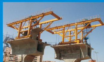
SE型节段梁架桥机在印度施工 SE type Segmental Beam Erector construction segment in India.jpg
