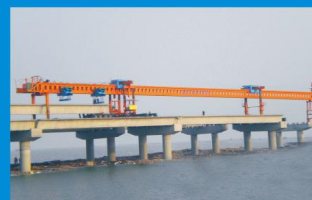
DJ型单导梁架桥机在天津滨海大道架桥施工 DJ-type Single Guided Beam Erector in Tianjin Binhai Avenue bridge construction
