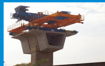
SE型节段梁架桥机在马来西亚施工 SE-type Segmental Beam Erector construction in Malaysia
