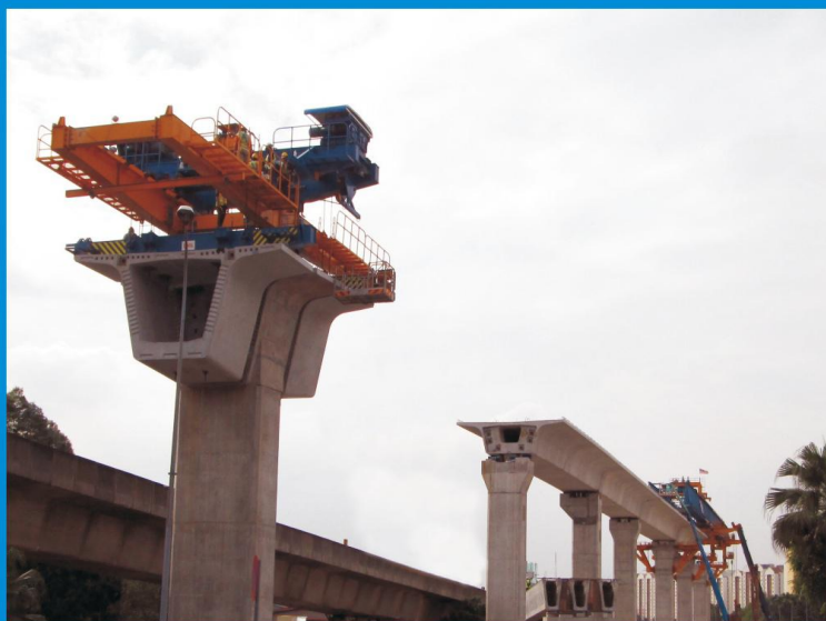
SE型节段梁架桥机在印度施工 SE type Segmental Beam Erector construction segment in India.jpg
