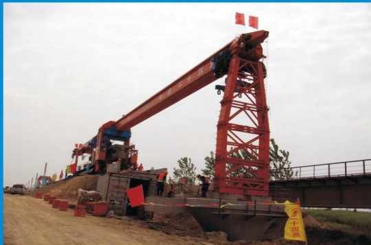
DJP200型铁路架铺机在宁启铁路架梁施工 DJP200 model track layer in Ningqi girder railway construction
