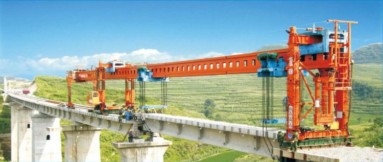
DJ型公铁两用架桥在尼日利亚架梁施工 DJ-type dual function girder erection machine in Nigeria
