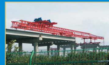
双导梁架桥机在慈利架桥施工 Double Truss Beam Erector machine construction in Cili District Hunan
