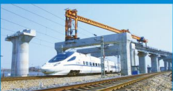
跨铁路线架梁施工 Girder across railway construction
