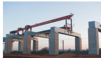
DJP180型铁路架铺机在内蒙古架梁施工 DJP180 Series Track Layer erecting a bridge in Inner Mongolia
