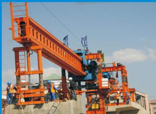
DJ型单导梁架桥机在埃塞俄比亚架设轻轨梁 DJ-series Single Box Girder Beam Erector has erected U shaped rail beams in Ethiopia
