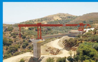
DJ型单导梁架桥机在希腊架梁施工 DJ-type Single Guided Beam Erector in Greece bridge construction
