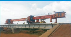
架桥机桥间转移 Transfer bridge between erecting machine
