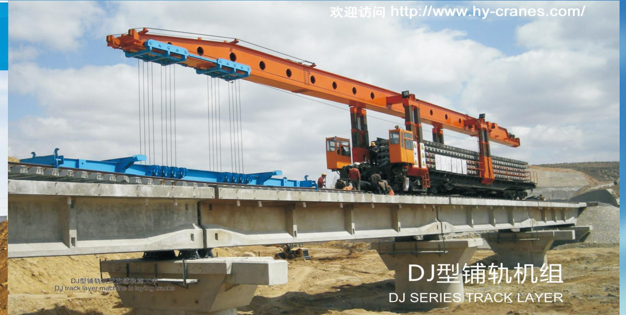
DJK166型铁路架桥机在兰渝铁路架梁施工 DJK166 Railway Beam Erector is working at Lan-Yu Railway construction
