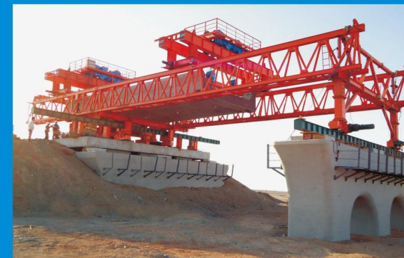
JSHB型双导梁架桥机在兰新二线架设重240吨的“U”型铁路梁 JSHB Double Truss Beam Erector -Lanzhou-Xinjiang Second Link Rail Road, 240 tons of U shaped rail beam
