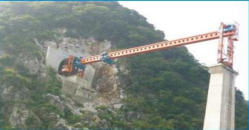
出隧道口架梁施工 Girder construction of the tunnel
