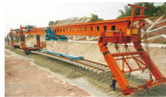
DJP180型铁路架铺机线路铺轨 DJP180 Series Track Layer laying railway track
