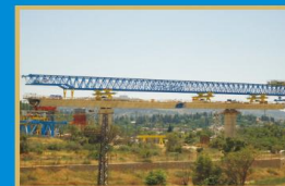
整孔合拢 Span closure
