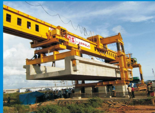
DJ型单导梁架桥机在印度架设重280吨的铁路轻轨“U”型梁 DJ-series Single Box girder Beam Erector has erected 280 tons of heavy rail light rail U shaped beam, India project
