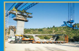
桥下提梁 Segment lifting under the bridge
