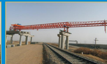
双导梁架桥机在天津滨海大道架桥施工 Double Truss Beam Erector in Tianjin Binhai Avenue bridge construction
