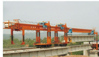
DJP180型铁路架铺机在重庆架梁施工 DJP180 Series Track Layer erecting a bridge in Chongqing
