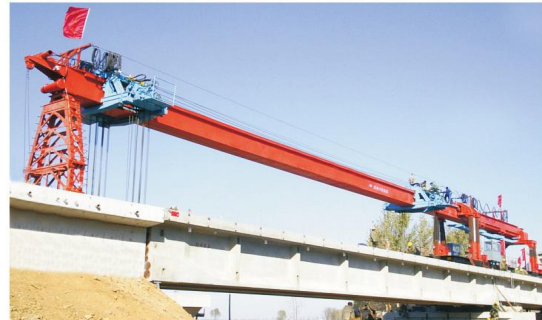
DJK166架桥机在南疆铁路架梁施工 DJK166 Railway Beam Erector is working at Nanjiang Railway construction
