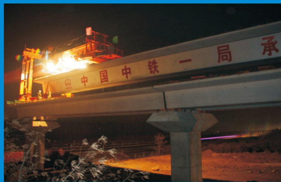
DJ型单导梁架桥机在印度架设“U”型轻轨钢梁 DJ-series Single Box Girder Beam Erector has erected U shaped rail steel beams in India
