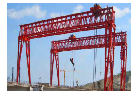
Beam lifting gantry crane
